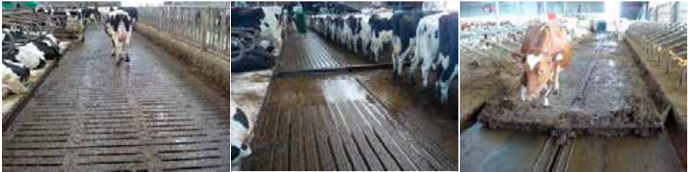
Fig. 1: Floor types in the field survey. Left: slatted floors (SFR and SFL). Centre: grooved floor (GF). Right: V-shaped asphalt floor (AF) (© D. Snoek)
