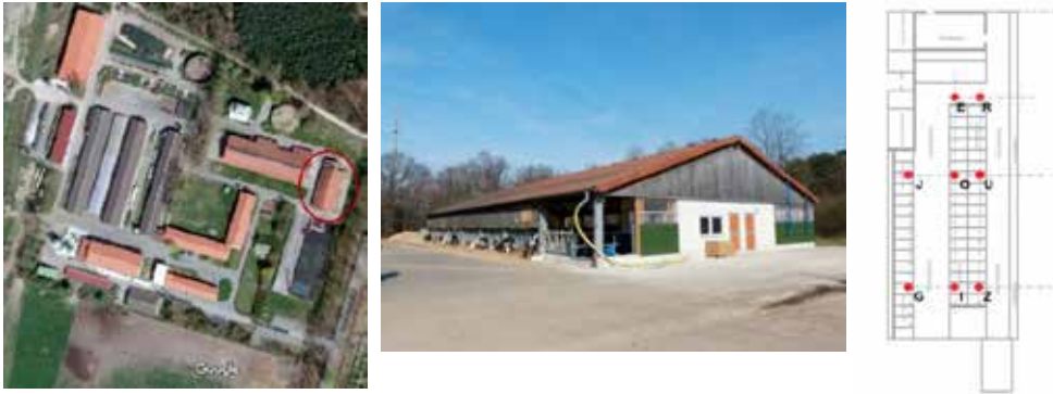
Abb. 1: Milchviehstall in Groß Kreutz, Deutschland. Lageplan (links) (© Google maps), Ansicht aus Hauptwindrichtung (Mitte) und Verteilung der Temperatur-Feuchte-Sensoren (rechts) (© ATB) Fig. 1: Dairy barn in Groß Kreutz, Germany. Map of the farm (left) (© Google maps), photograph of the barn viewed from the main prevailing wind direction (middle) and layout of the barn and sensor positions (right) (© ATB)
